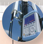
Network rollout and commissioning
